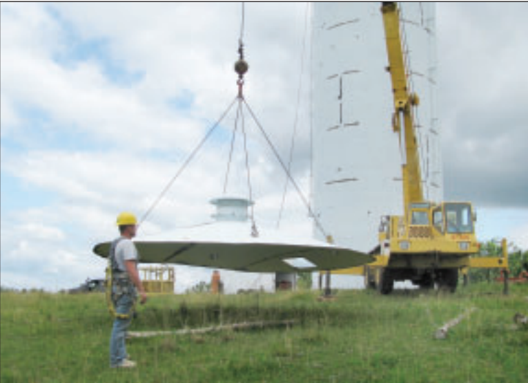
PHOTO BY DARYL K. TABOR After nearly 25 years of towering over the Crayne landscape, an 80-foot tall water tank used by Crittenden-Livingston Water District met its end this week at the hands of a crew from Preferred Tank & Tower Inc., of Henderson. Work to remove the 200,000-gallon tank began weeks ago, but foreman Danny Loveless (top left) and Brandon Miller climbed atop the tower last Thursday with cutting torches to make the final cuts for a crane to remove sections. After the cap was removed (above and right), nine separate ringed-sections were lifted one at a time and hauled away. District Superintendent Donnie Beavers said the tank was obsolete and the $7,500 removal cost was a far better option than the $60,000 estimate to have the standpipe tank painted.
